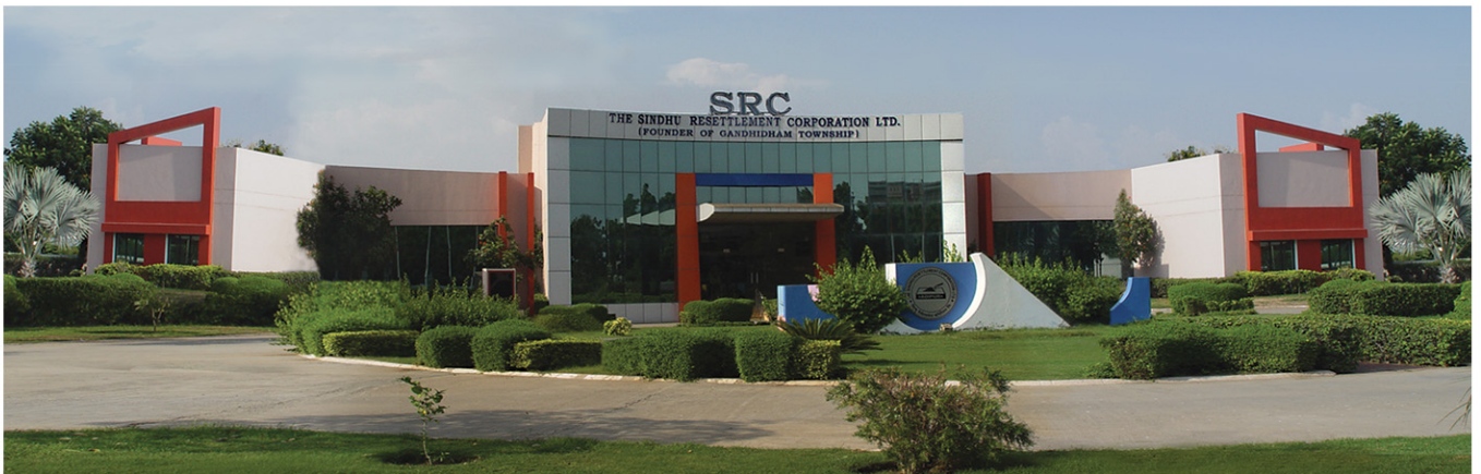
Headquarters of Sindhu Resettlement Corporation Limited at Adipur (Kutch)
